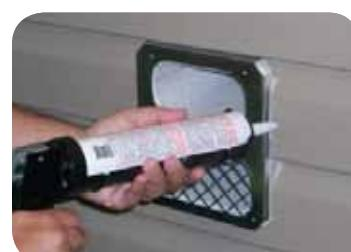
**NOTE :** Seal the perimeter of the connector plate using exterior rated multi-use silicone sealant.
