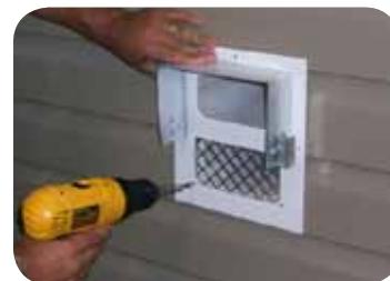
Attach the face plate to the transition portion as shown using (4) #10 x  $\frac{5}{8}$ " screws, then using the (3) #10 x 2" screws, fasten to the exterior wall.
