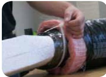
Secure the vinyl duct to the insulated transitions portion using the provided tie wraps.
