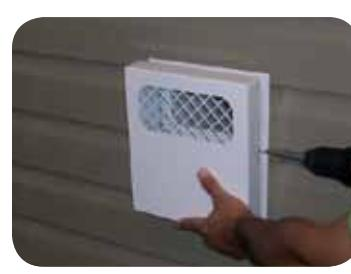
Secure the ventilation cap by fastening it to the face plate using the (4) #10 x  $\frac{5}{8}$ " screws.
